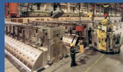
Cooling of aluminum smelters
